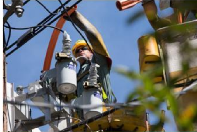
Electric Upgrades by Town
