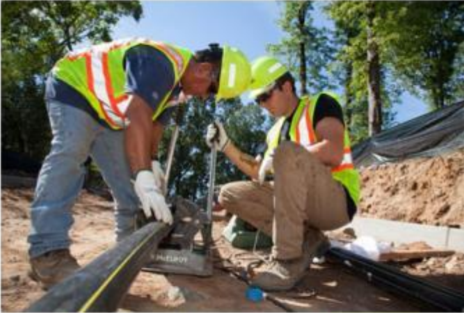
Gas Main Replacement by Town
